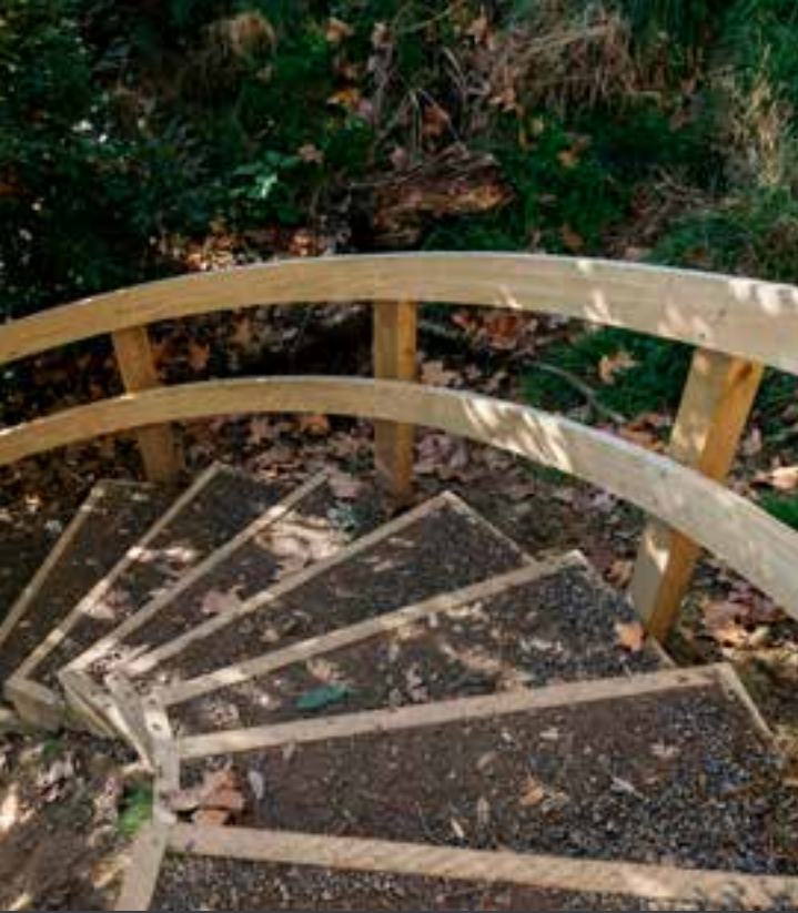
New stairway and handrail, Ōhinerau / Mount Hobson
